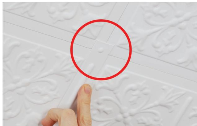
While not necessary for many installations, a few dabs of adhesive can be added to each of your strips before installing. This adds an extra layer of security and increases the durability of your installation.
