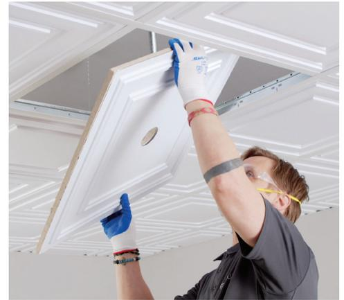
If you are using a refacing style with a mineral fiber backing panel above it, per IAPMO UES Evaluation Report 310, sprinklers must be located a maximum of 3 in. below the ceiling grid, and sprinkler pass-through holes must be 0.25 in. smaller in diameter than sprinkler trim rings/escutcheons/cover plates.
