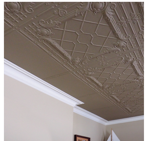
High-relief ceiling elements can be bordered with low-relief elements to simplify perimeter conditions. Crown moldings can complement the ceiling style and embellish the wall-ceiling intersection. Decorative strips can be used to cover suspension grid tees or the butt joints between tiles. Photo: Ceilume
