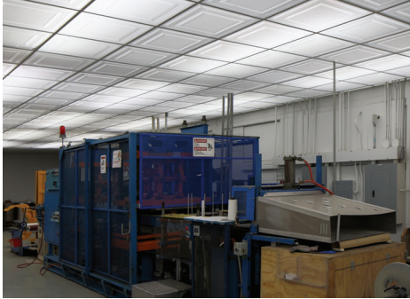
The factory's luminous ceiling provided even illumination and reduced noise. It also cut energy consumption because only the work area is heated or cooled, not the high-bay area above. Photo: Ceilume
