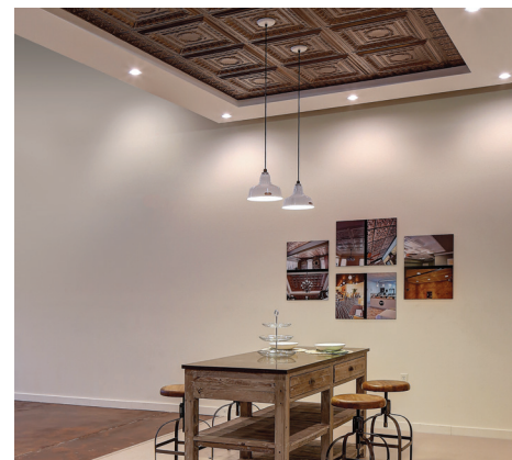
Faux finishes have expanded the aesthetic range of thermoformed ceilings. The wood-look (top) is used in 2 x 4 foot panels with staggered joints to suit a casual workroom. The metal-look (bottom) is neatly framed within a ceiling tray (soffit). It is difficult to distinguish the facsimiles from the original materials when seen at normal viewing distances. Their relative economy, ease of handling, and light weight, however, will be immediately apparent to installers. Design: Emma Davis / Photo: Ceilume
