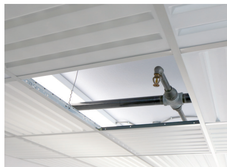
These translucent, drop-out ceiling panels were installed beneath existing strip lights and fire sprinklers to reduce remodeling expenses. Photo: Ceilume
