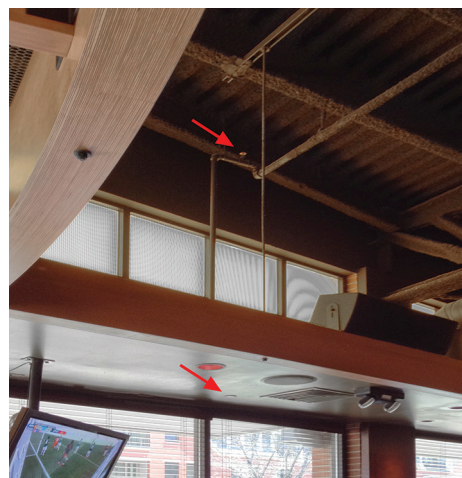
Sprinklers may be required both above and below soffits and ceiling clouds (see arrows). With drop-out ceiling panels, however, one set of sprinklers above the ceiling may be sufficient. Photo: Ceilume
