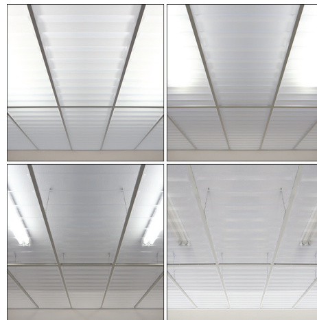
Translucent panels (top left) create the most even light distribution. Frosted panels (top right) hint at what is above the ceiling. Transparent panels fully disclose what is above the ceiling whether above-ceiling lamps are on (bottom left) or off (bottom right). Each ceiling style will scatter light differently; some display patterns of highlights and shadows or sparkling refractions that become animated as one moves through a room. Photo: Ceilume
