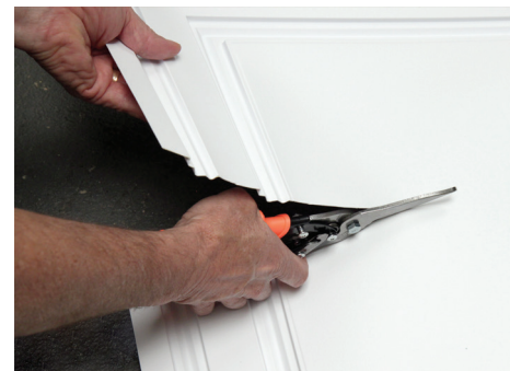
Lightweight and easy to install, thermoformed panels and tiles can be trimmed with scissors or aviation snips. Although the products are made with thin material, panels and tiles are robust, do not release fibers, and are not frangible. Photo: Ceilume
