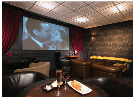
Ceiling panels with classic detailing complement the theme of the moving screening room in a Noir Lounge in San Francisco. The thermoformed translucent material "creates a gentle glow and avoids glare on the screen," according to Gi Paoletti of G. Paoletti Design Lab. She adds that dimmable LED lamps above the luminous ceiling avoid the need for pendant light fixtures that would block patrons' view. Design: G. Paoletti Design Lab / Photo: Stuart Locklear
