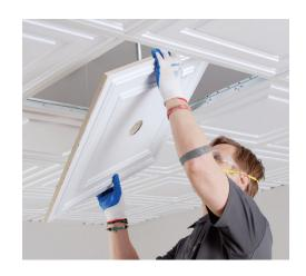
If you are using a refacing style with a mineral fiber backing panel above it, per IAPMO UES Evaluation Report 310, sprinklers must be located a maximum of 3 in. below the ceiling grid, and sprinkler pass-through holes must be 0.25 in. smaller in diameter than sprinkler trim rings/escutcheons/cover plates.
