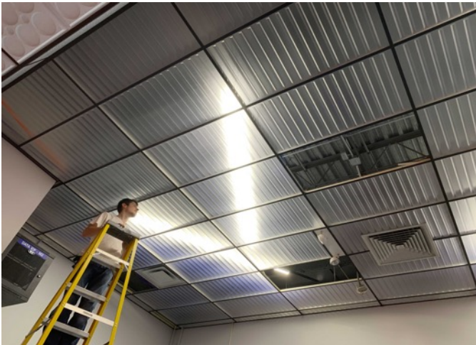
Left: Visual excitement was generated in the elementary school by arranging the new LED fixtures in zigzags above frosted ceiling panels. Installation of the lightweight thermoformed panels was performed by staff. Right: Clear panels in the middle school computer lab allow views of above-ceiling mechanical equipment and structural members, a metaphor for the computer “architecture” and an invitation to students to expand their creative vision.
