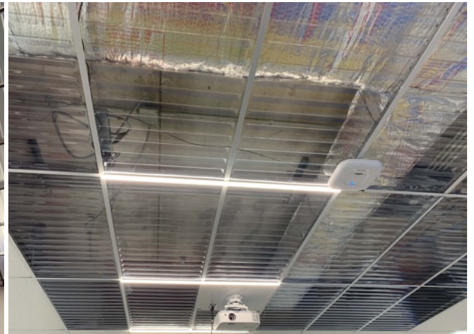
Left: Visual excitement was generated in the elementary school by arranging the new LED fixtures in zigzags above frosted ceiling panels. Installation of the lightweight thermoformed panels was performed by staff. Right: Clear panels in the middle school computer lab allow views of above-ceiling mechanical equipment and structural members, a metaphor for the computer “architecture” and an invitation to students to expand their creative vision.
