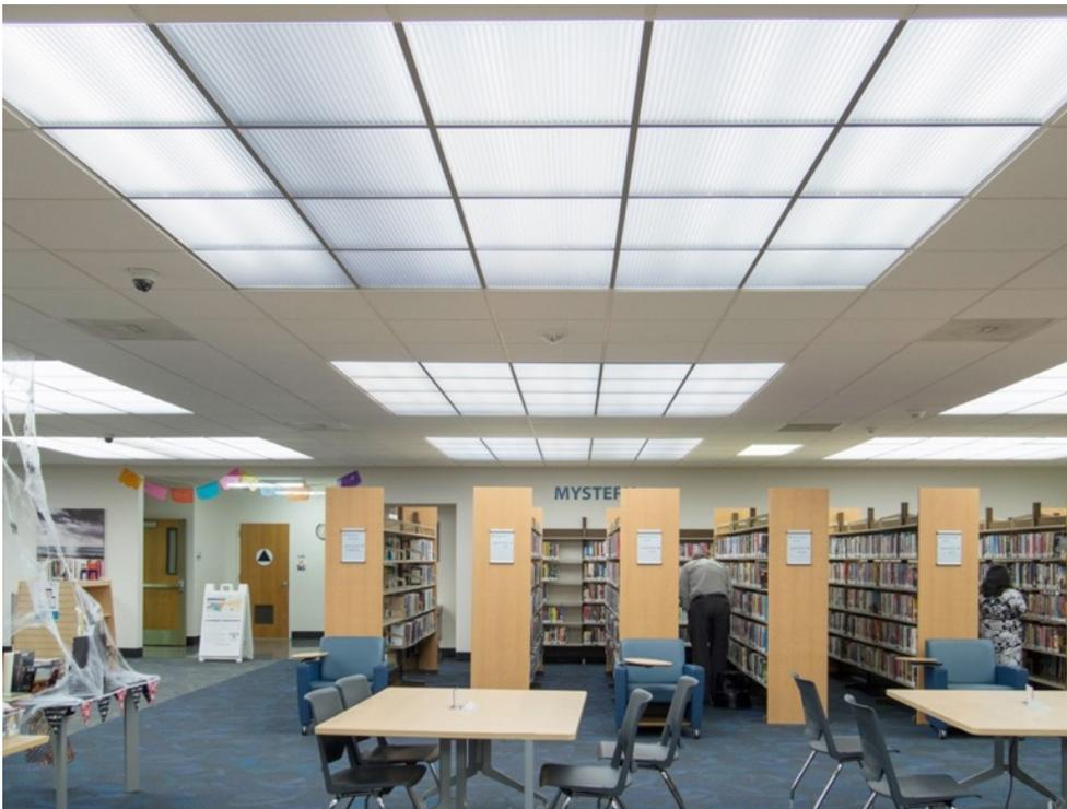
**Replacing the aged, yellowed lenses of the luminous ceiling with new, thermoformed light-transmitting panels markedly increased illumination in both library branches. The later switch to LED lamps improved the lighting further while lowering energy consumption.**
