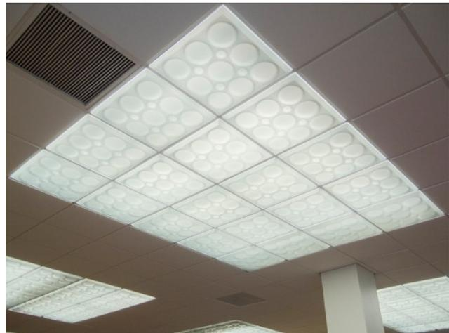
**RIGHT: New thermoformed panels, like the Roman Circles style that were used at the Sunkist branch, were dropped into the existing support grid.**
