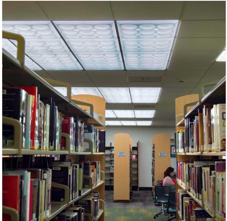
**LEFT: Old fluorescent tubes were replaced with energy-conserving LED tubes. New high-efficiency ballasts had to be installed, but that allowed the library to keep the existing fixtures and light boxes and minimize the upgrade cost. (Photo courtesy of Anaheim Public Library)**
