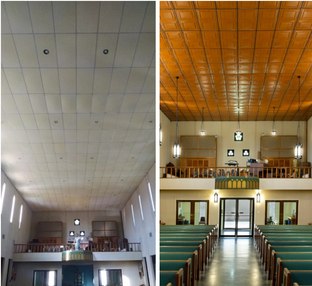
Left: The old ceiling had sagging, mineral fiber panels that had been badly stained by water from roof leaks and by incense used in the worship. (Photo courtesy of the Church of St. Mary the Virgin) Right: The new, thermoformed ceiling is stain resistant, washable, and impervious to water. (Cropped from posted image.)
