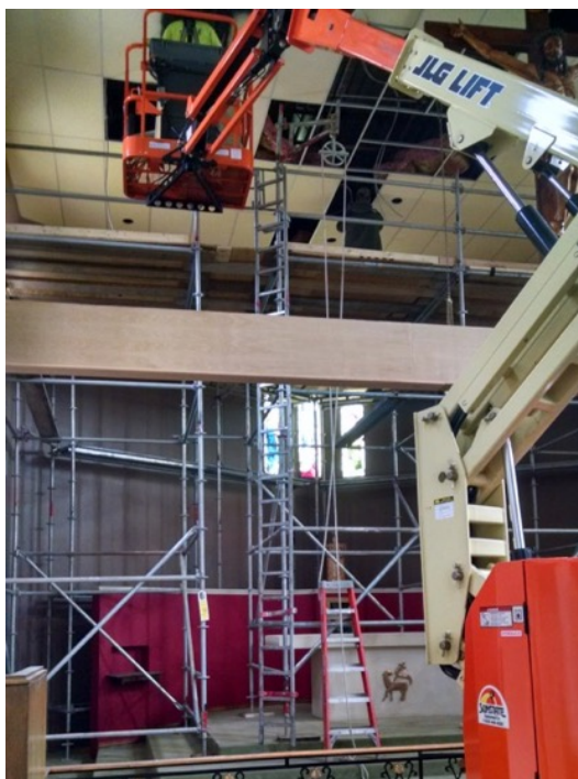
Left: Above the new baptismal font, a border of the original, water-damaged mineral fiber ceiling had not yet been replaced when this photo of the new baptismal font was taken.
