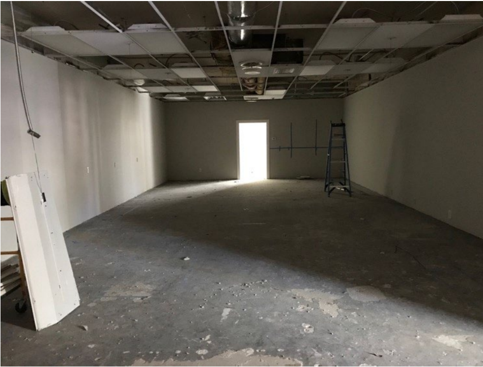
Before renovation, the ceiling was in in bad shape, with a warped grid and many missing panels. Replacing the grid proved inexpensive, and the owner was glad to be rid of the old flat ceiling tiles.
