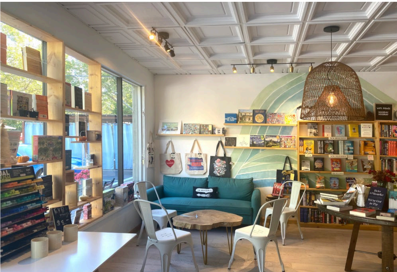
Border panels at the edges of the ceiling are a different pattern, Oxford, a shallower concentric square that mirrors the coffers but presents a profile that is more visually appealing when cut at the edges of the ceiling. Cutting is easy with a pair of snips.
