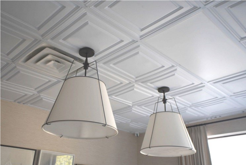
Yellowed T-bar grids were re-faced with Ceilume's EZ-On Drop Ceiling Grid Covers that quickly snap onto existing grids.
