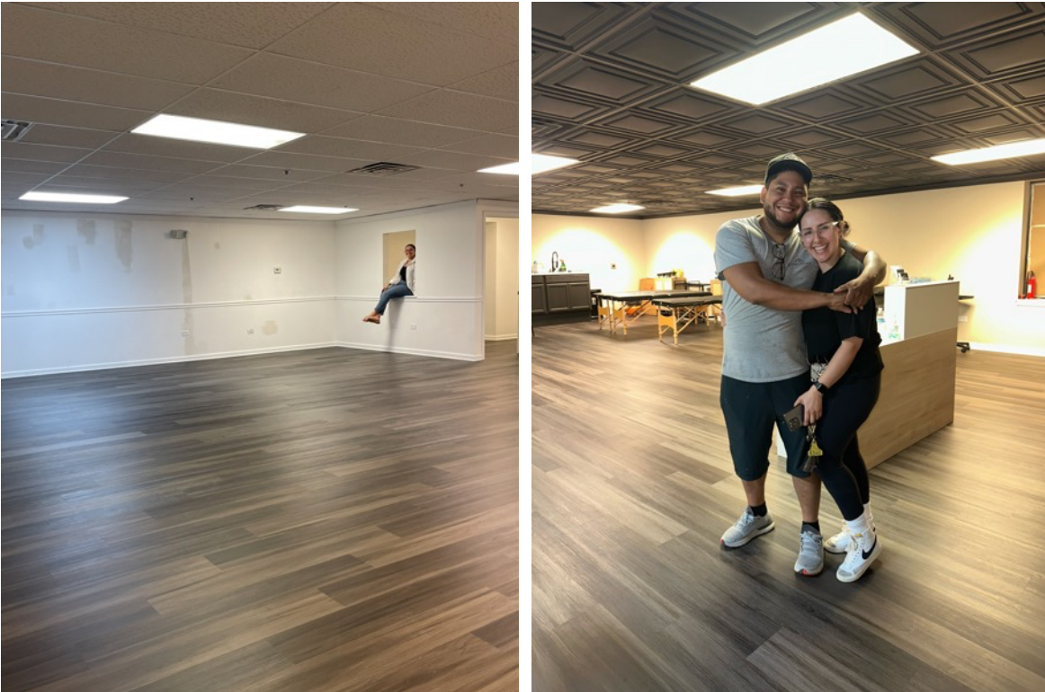
The old ceiling – mineral fiber acoustic tiles – was the only major element that Lorena Perez felt needed to be changed when she took over her new business space. She and her husband, Rafael Abrego, installed the new ceiling themselves.
