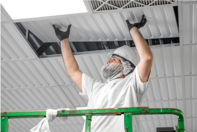
Thermoformed panels are lightweight, robust, and easy to install. They do not release fibers or other contaminants when handled to service above-ceiling equipment.
